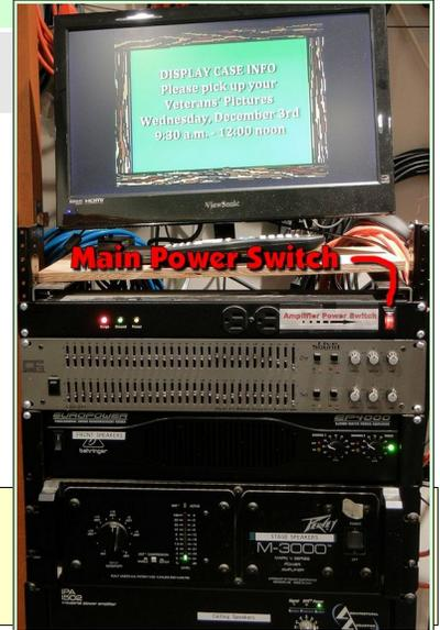
**NOTE:** If cameras or other video is being used, turn on the V-800HD first and wait until all lights stop flashing before turning on other video equipment.
